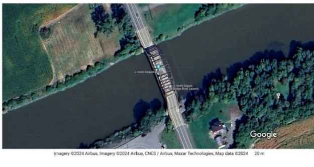
Figure 1: Overview of the J. Henri Séguin Bridge
